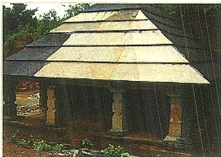
Jain Basadi Haduvahalli After Restoration
