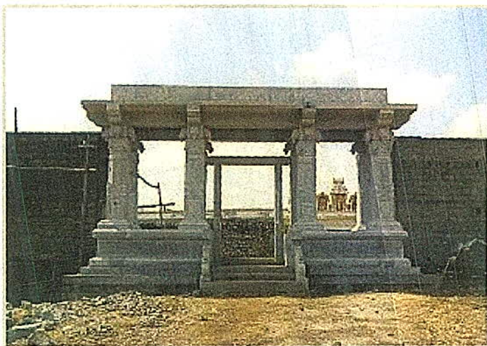
Kanakgiri Kshetra after Restoration
